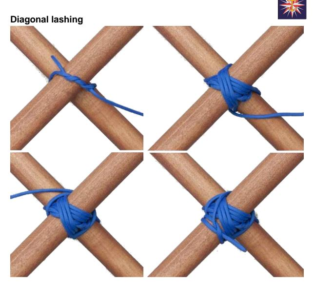
The diagonal lashing is binds two poles in a cross diagonally at 90° or 45°. Start with a timber hitch around the poles to secure the rope onto the pole. Make three turns in each direction - tightening steadily throughout the turns. Make two frapping turns, tightening the joint as much as is possible. To complete make two half hitches clinched into a clove hitch.
